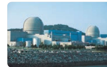
Nuclear Power Plant
