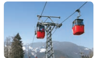
Cable Car Propulsion Rope
